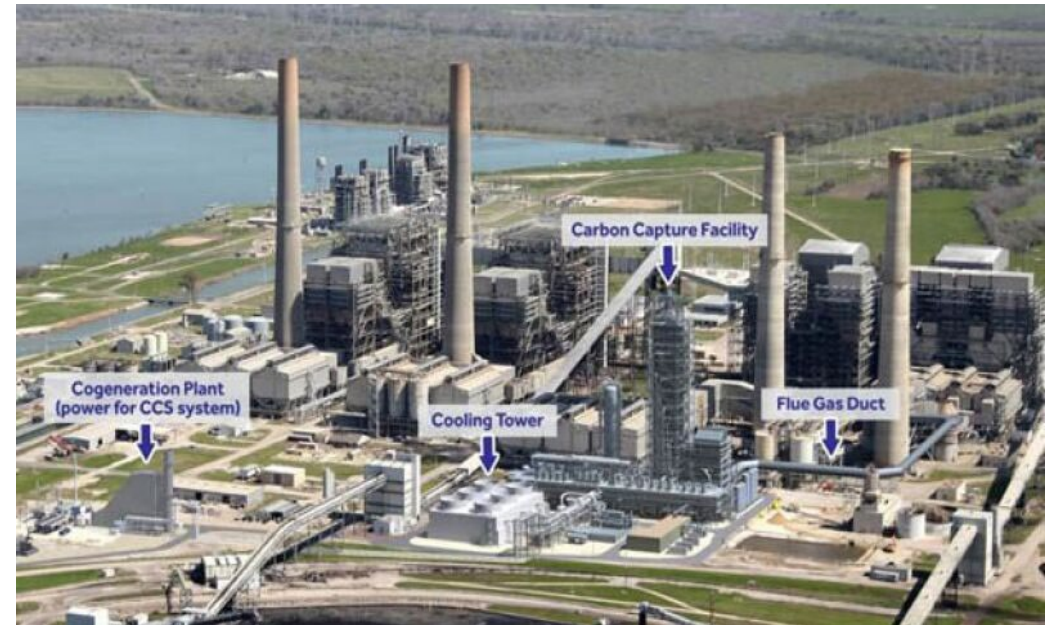
Carbon capture facility (coal plant) at the Petra Nova facility near Houston (1.4 mtpa target)
